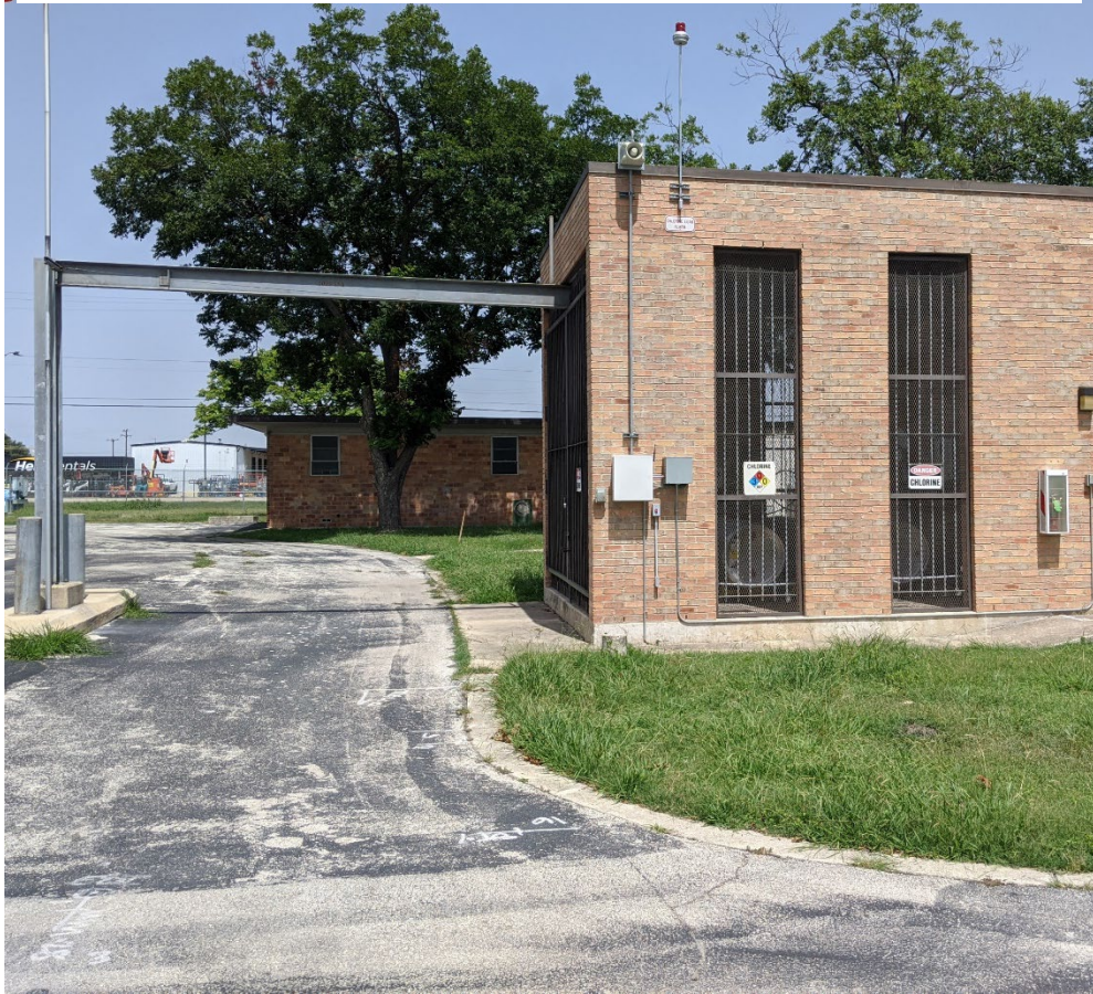
Existing gas chlorine building (demolish)
